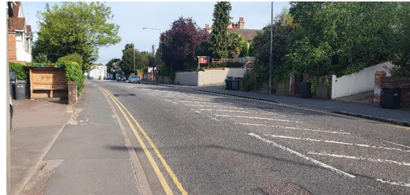
Figure 30: A40 London Road (existing)
